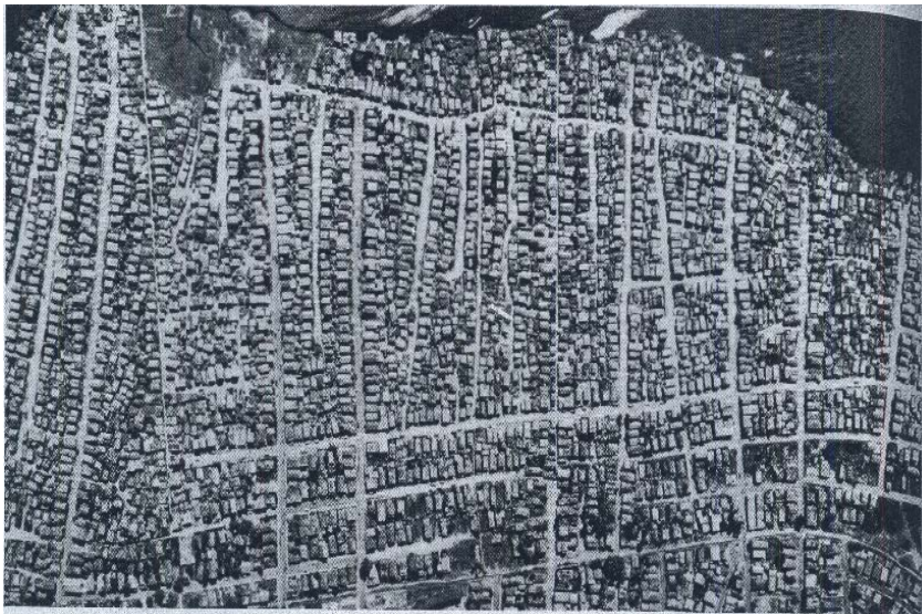
SAN JUAN SLUM AREA in the Santurce district sprawls along the edge of the tidal inlet (top) that connects the city's harbor with San José Lake. Ricketty buildings have been erected on stilts be-
